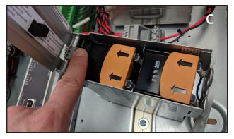
Once the UPS battery case is open, locate the fuse holder, towards the bottom left of the battery enclosure, and insert the fuse.
