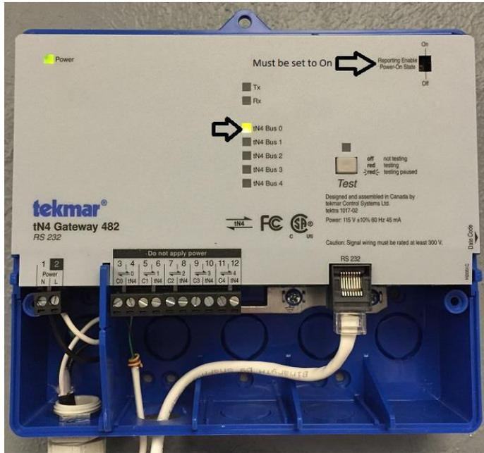
1. The LED that is 'ON' for Bus 0,1,2,3,4 is the 'PORT' number for you thermostats. If there are no LED's on, there is no communication on the tekmar tN4 network.
